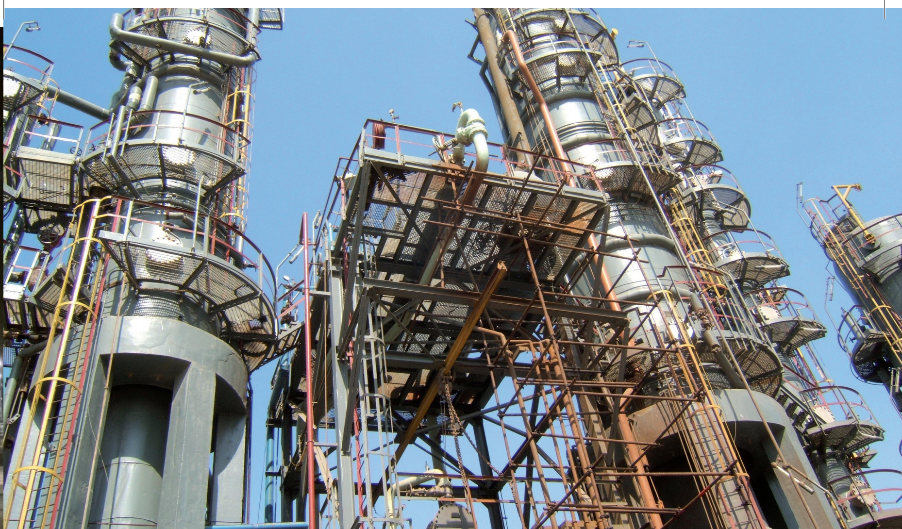
PROGETTO FEED PER LA NATIONAL REFINERY LTD., KARACHI (PAKISTAN). CRUDE AND VACUUM DISTILLATION UNIT REVAMPING. CAPACITÀ: 60.000 BPSD
