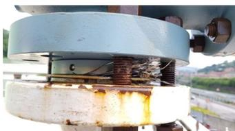
Figure 2: Damaged spiral.
