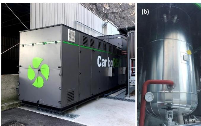
Figure 2: (a) C700 plant container; (b) C700 HTC jacketed reactor vessel
