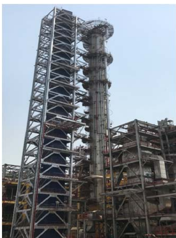
Figure 8: A Top DWC in an ISOM Unit in operation at BPCL Refinery (Mumbai, India).
